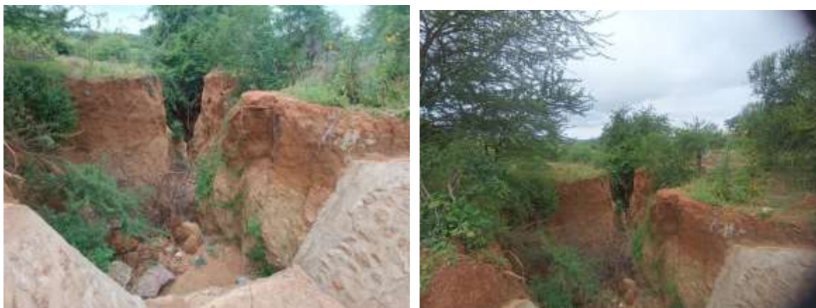
Figure 31: Gully due to improper disposal of road side water (Lat 0° 46' 29.6"s Long 38° 5' 36.2" E alt 992m)
