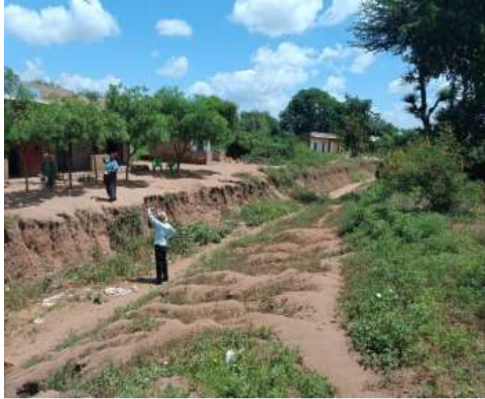
Figure 24: Huge gully dividing market center (Lat 1°2'40.4"S Long 38°11'
