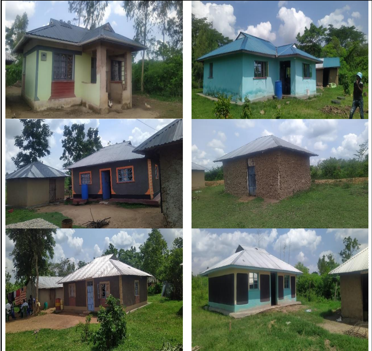
Figure 2-1: PAHs newly constructed residential structures
