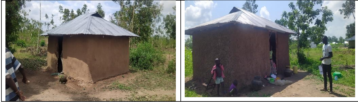
Figure 2-3: PAHs newly constructed residential structures
